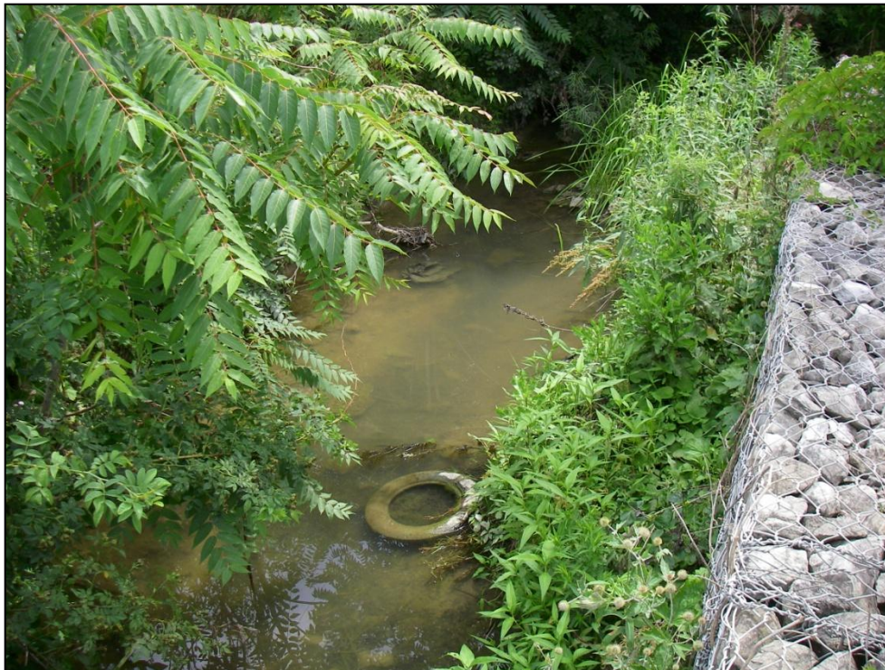
Photo 18: Wolfe Drain looking southeast (upstream) from Howard Avenue.
