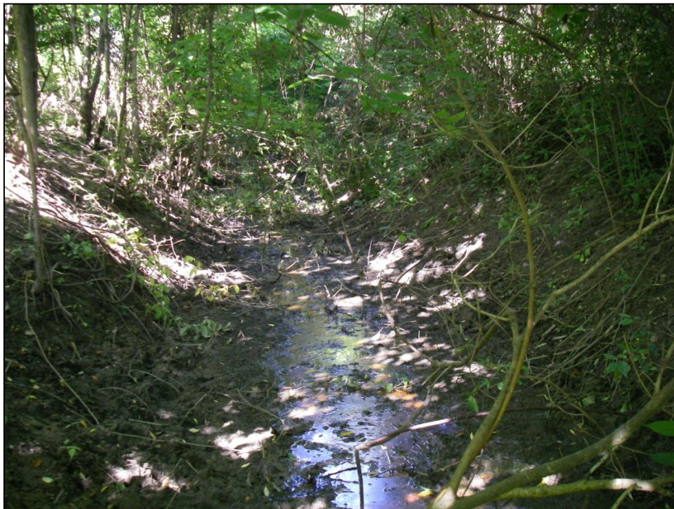
Photo 6: Youngstown Drain, looking southwest (downstream) from the E.C. Row Expressway to Huron Church Road eastbound to southbound off ramp culvert. Note the oily sheen on the surface.
