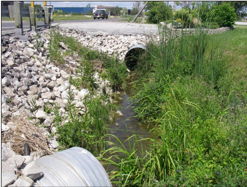
Photo 19: Wolfe Drain looking east (upstream) from the Talbot Road/Outer Road intersection.
