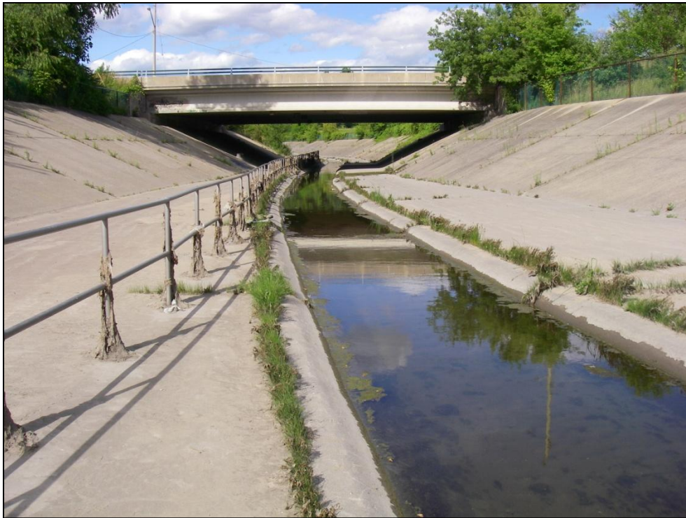
Photo 7: Turkey Creek, looking northeast (upstream) towards Huron Church Road.
