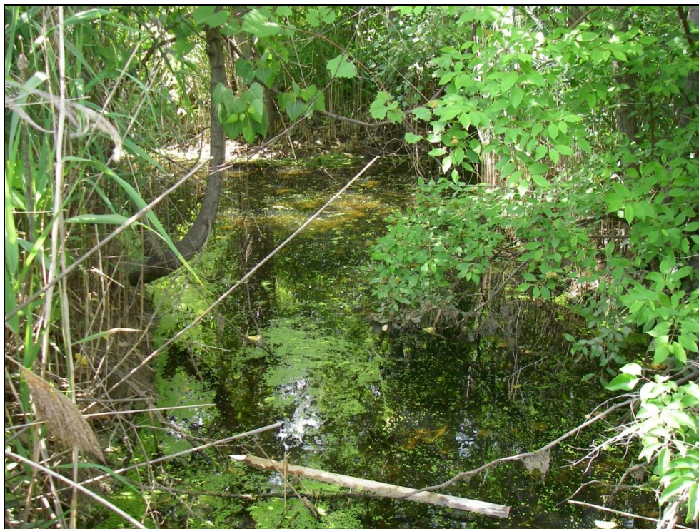
Photo 2: McKee Drain, looking northwest (downstream) from the E.C. Row Expressway culvert crossing.
