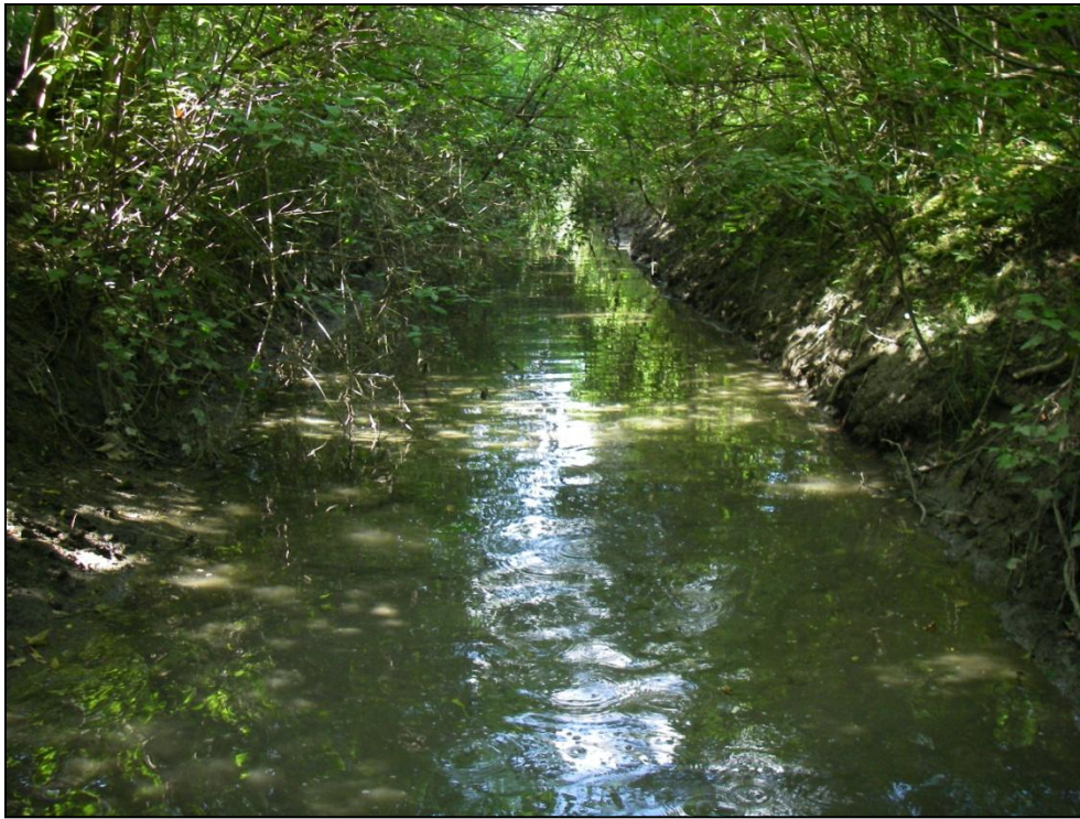
Photo 3: Basin Drain, looking north (upstream) towards the E.C. Row Expressway crossing.
