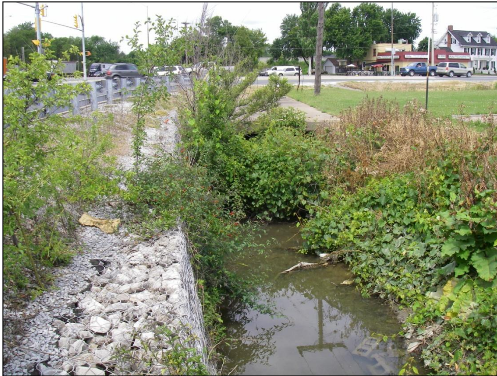
Photo 17: Wolfe Drain looking northwest (downstream) towards Howard Avenue.
