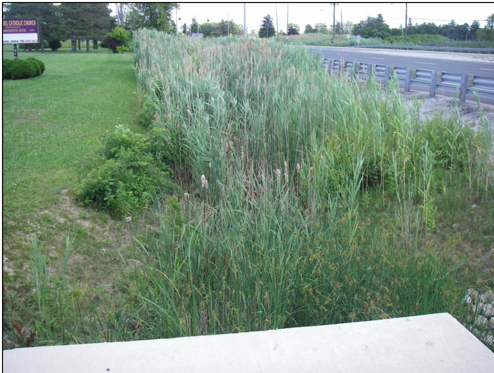
Photo 20: Collins Drain looking south (upstream) from the Talbot Road/Outer Road intersection.
